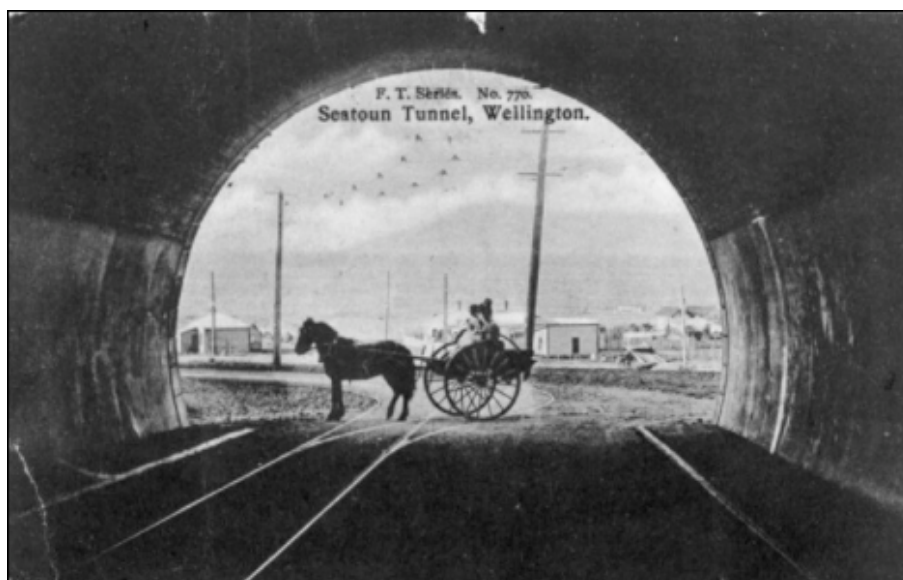
Figure 10 The new tram tunnel to Seatoun, ATL, ½-091609-F
