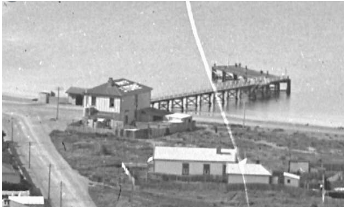
Figure 14 Seatoun wharf 1916, showing cross bracing of the approach wharf, the tea rooms, changing shed and shelter, ATL 1/4-018521-G
