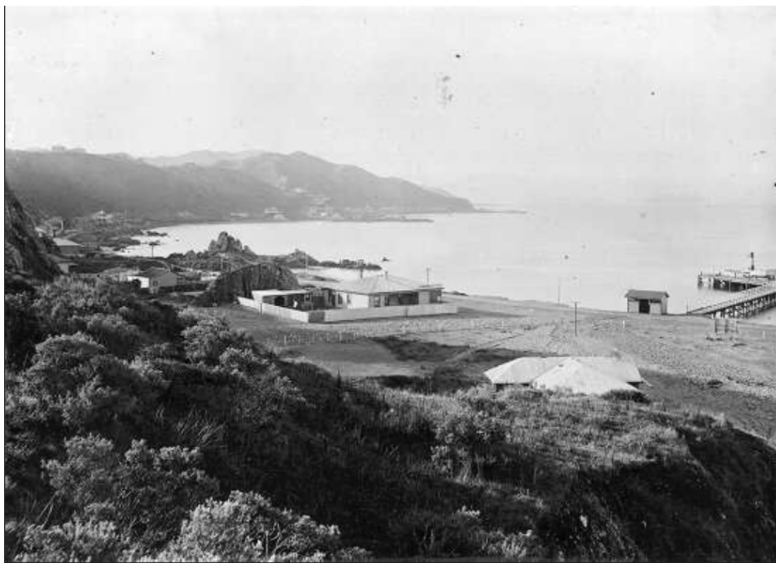
Figure 15 Wharf showing newly built passenger shelter, 1904, PAColl-7489-95
